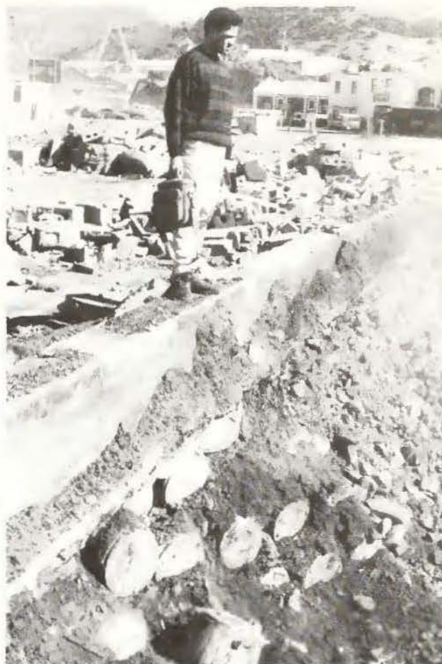
Fig. 6. Photograph depicting A part of the breakwater feature, constructed in one section of concrete barrels and filled with stone and yellow clay at the other end.
